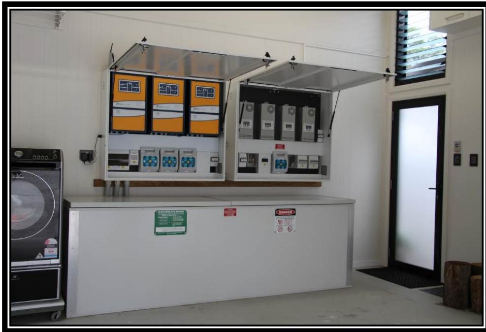
Figure 3. Residential 3 Phase Energy Storage System
