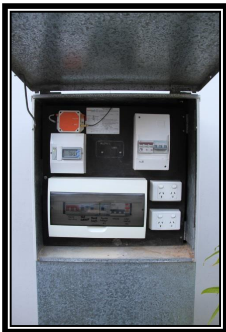
Figure 4. Customer's meterbox
